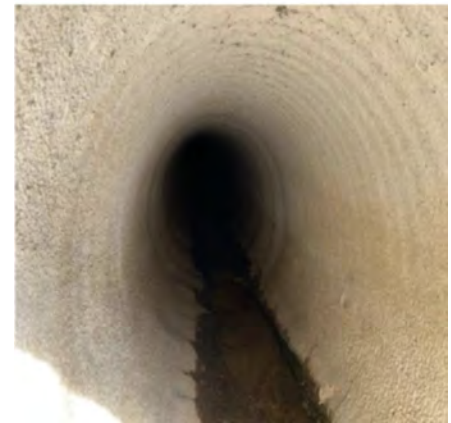
Pipe re-lining completed for Colorado DOT 2004
